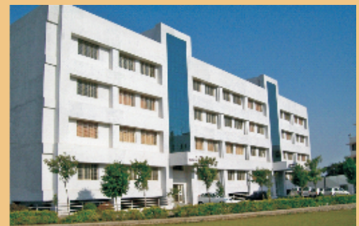
Building of Mechanical Department
