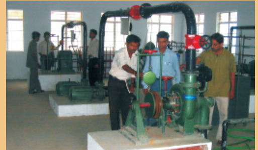
Fluid Machinery Laboratory
